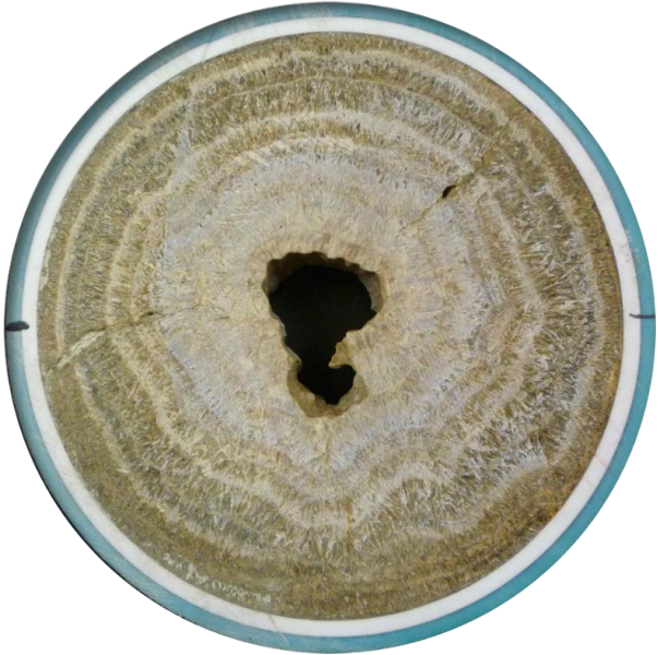
OPERATIONAL ISSUES WITH STRUVITE BUILDUP
